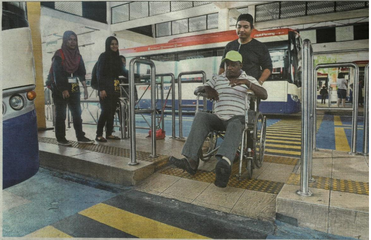
Sloped platforms make it possible for wheelchair users to cross bus lanes but the hand railings on this tactile pavement are an obstruction to the blind.
