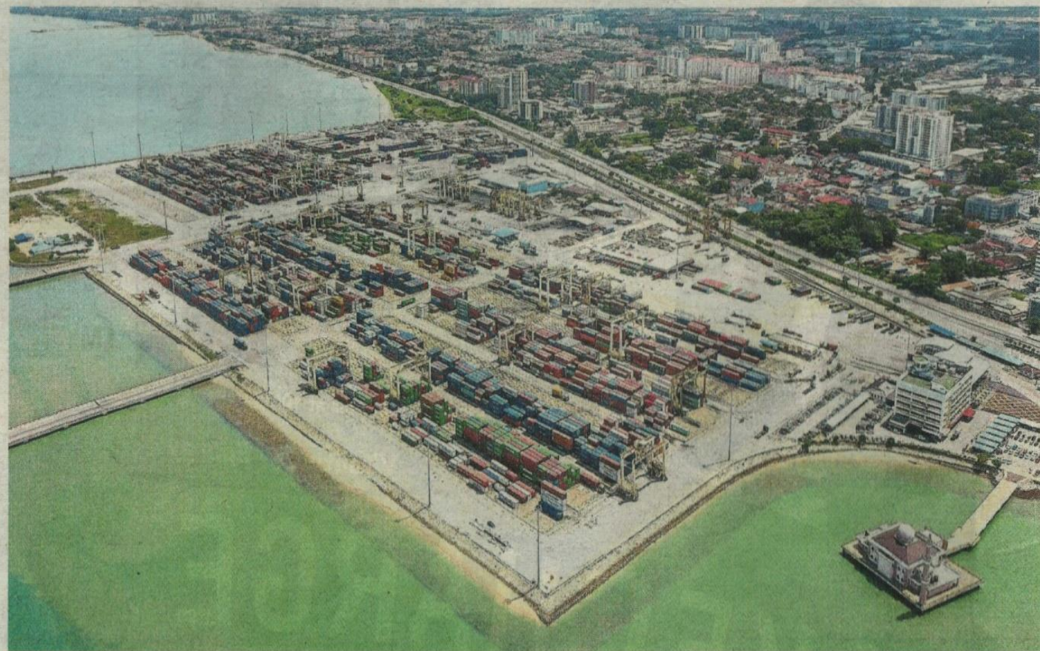
Revamp underway: An aerial view of NBCT in Butterworth, Penang.
