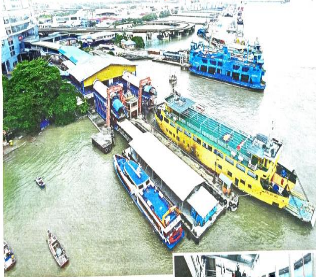
Entering new era: An aerial view of the Sultan Abdul Halim ferry terminal in Butterworth which will be upgraded soon. — CHAN BOON KAI and ZHAFARAN NASIB/The Star
